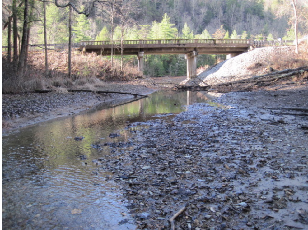
Photo 1. Downstream view of STR-2 (Maddens Branch) taken toward existing bridge
